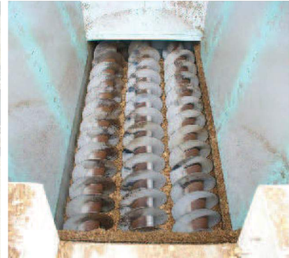
Mounting in discharge screw (wood-fired power plant)
