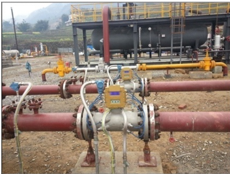
LYNSB-200mm PN6.3MPa application for shale gas distribution metering in Ning 201H1 platform in Sichuan gas field
