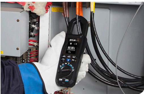
Verify amperage measurements
